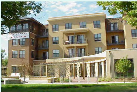
West River Commons Lake Street Corridor
